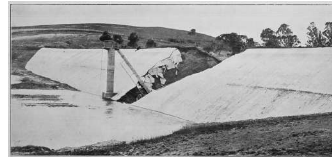
The collapse of the Marton water supply dam 1912.
